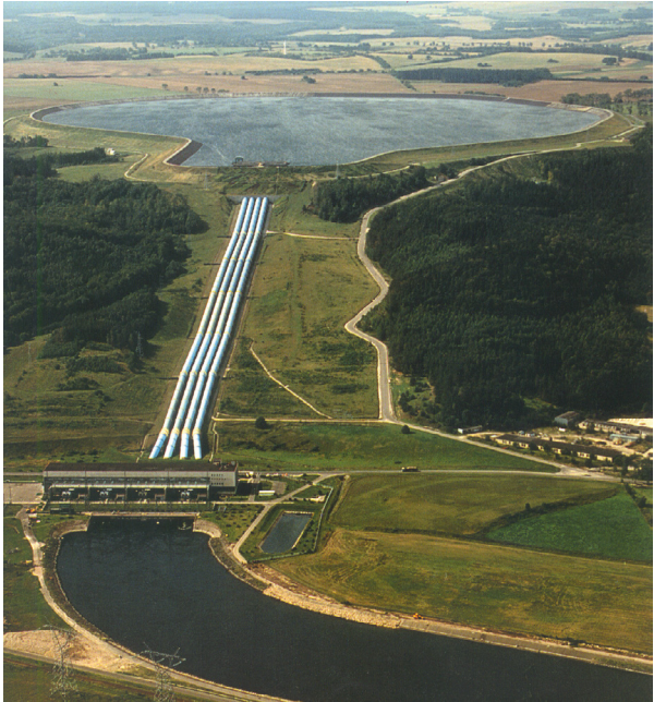
Fig. 3. The view of EPP Żarnowiec, conduits, and the upper reservoir.
