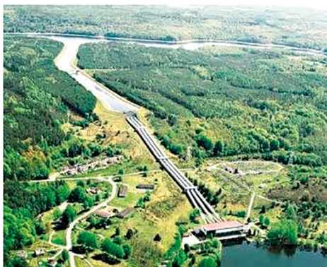
Fig. 4. The view of the power-plant Żydowo, pipelines, and open channel.
