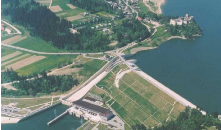
Fig. 6. The View of Solina Dam, upper reservoir, pumped-storage power-plant and lower reservoir Myczkowce.
