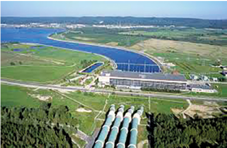
Fig. 2. The view of the part of conduits open channel and the Lake Żarnowiec.
