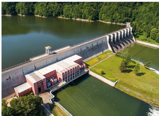
Fig. 10. The view of the dam and power-plant Rożnów.
