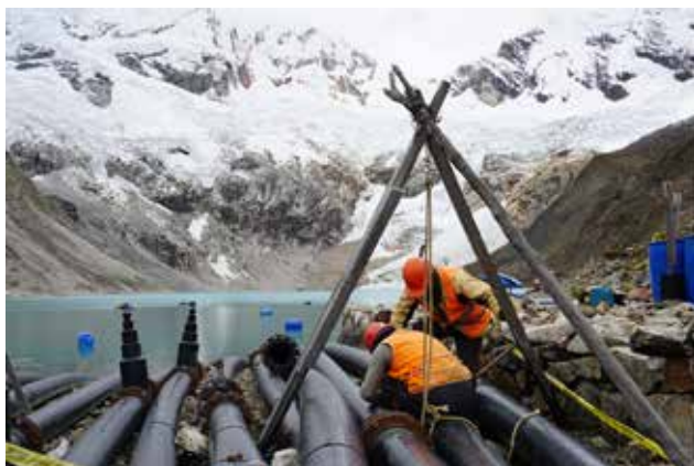
Figure 7. The Palcacocha Glacier lake (Peru) is drained using siphons to avoid Glacier Lake Outburst Floods (GLOF) (Photo: Christian Huggel)
