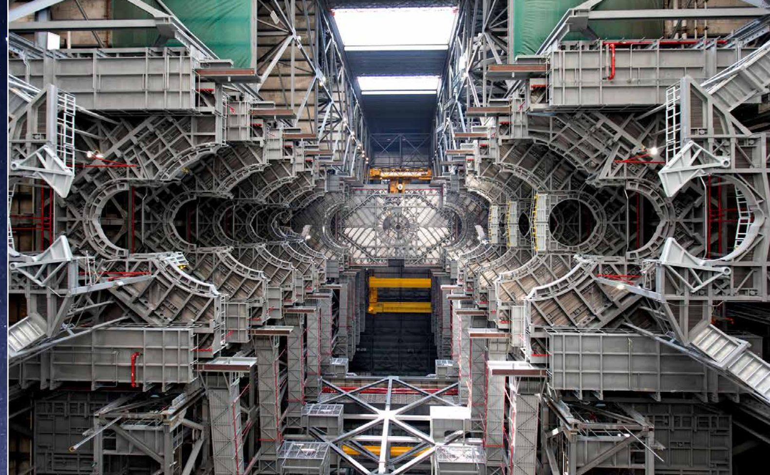
A view looking up at the 10 levels of work platforms in High Bay 3 inside the Vehicle Assembly at NASA's Kennedy Space Center in Florida. The work platforms will surround and provide access for service and processing of the agency's Space Launch System rocket and Orion spacecraft for Artemis missions. Photo credit: NASA/Glenn Benson
