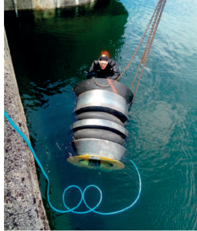
Fig. 4. Submersible closing facility during installation [PPH-1200 technical documentation; K+K servis Ltd.]
