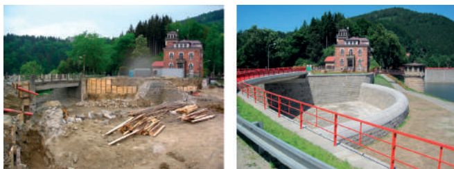
Fig. 11. WS Bystřička – safety overflow during and after reconstruction [photo by Hodák]
