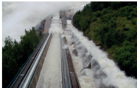
Fig. 2. WS Orlik – spontaneous outflows of ship lifts during the flood in August 2002 [photo by D. Richtr]
