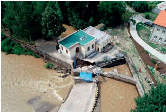
Fig. 7. An overall view on the collapsed weir
