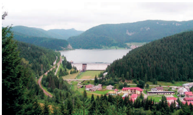
Fig. 1. Palcmanská Maša Dam situated in National Park – Slovak Paradise [photo by L. Uhorščák]
