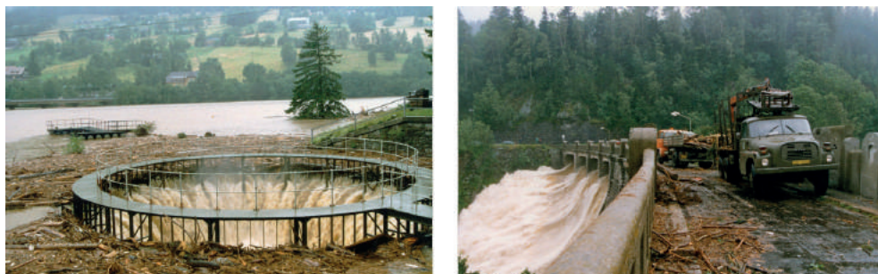
Fig. 7. WS Labská during the flood in 1997 – congestion of the shaft spillway, removal of sediments (floating debris) in front of the crest spillway [photo by Kyrián]
