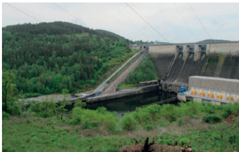
Fig. 15. WS Orlik – view of the dam, present state [photo by D. Richtr]
