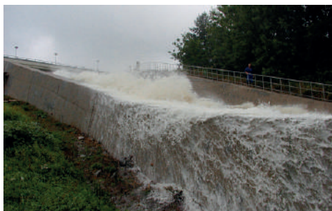
Fig. 3. WS Řimov – overflowed chute during the 2002 flood [photo by M. Sedláček]
