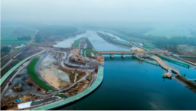
Fig. 7. Aerial view, Malczyce barrage, Poland
