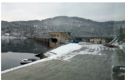
Fig. 17. WS Orlik – view of the inflow into the new spillway, the current state [photo by D. Richtr]
