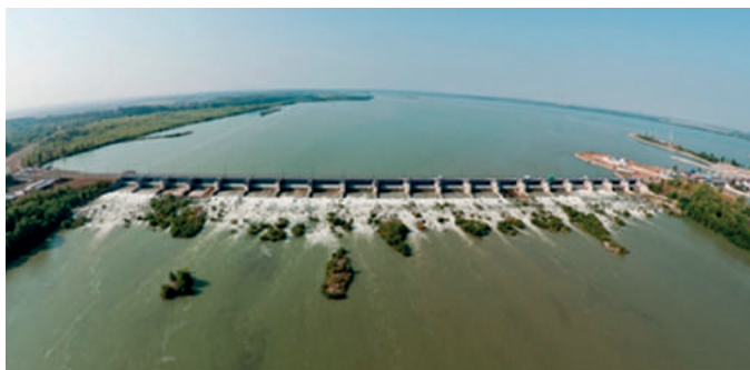
Fig. 5. Cunovo step – weir in inundation
