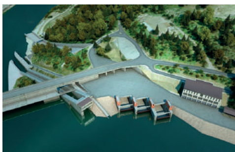
Fig. 18. WS Orlik – visualization of the new spillway, view of the inflow [Auquatis a.s.]
